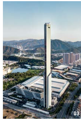
03 At 248 metres tall, the test tower of TK Elevator in the Chinese province of Guangdong is one of the tallest buildings in the world. The tower is used for high-speed tests and is designed for cableless elevator systems.
